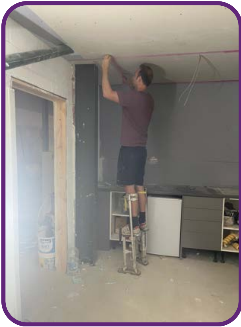
A huge thank you to Lee Town from Town Plastering for plastering the entirety of the extension!
